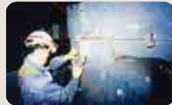
Installing fiber sensor on the motor of coal-mine shaft
